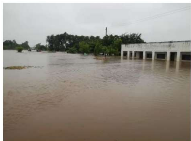
Flooding at Nkando bridge (14 March)
