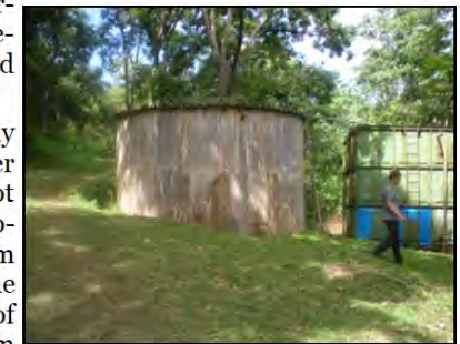
The existing water tank
